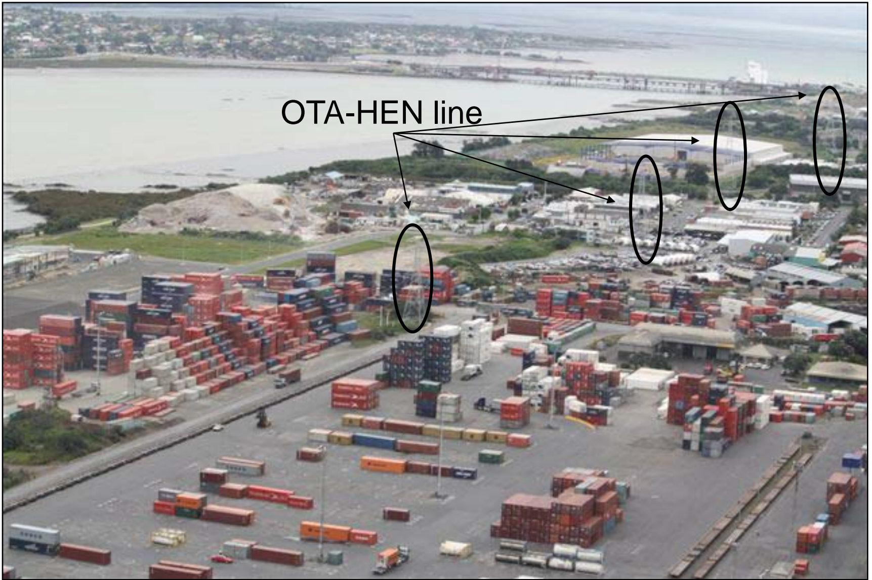
Metrobox container storage yard, Onehunga
