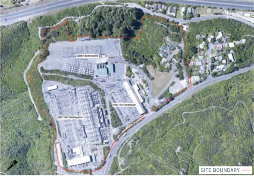
Existing Haywards → substation
