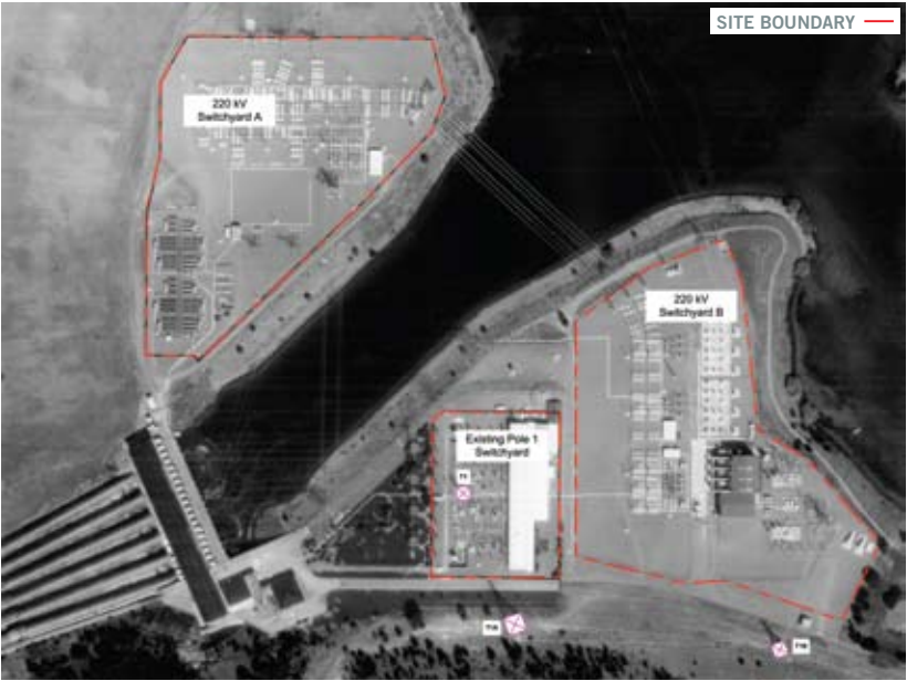
Existing Benmore → substation
