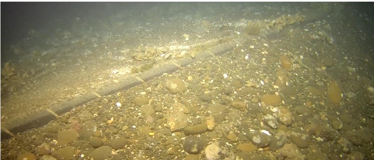
A HVDC cable on the sea floor of the Cook Strait
