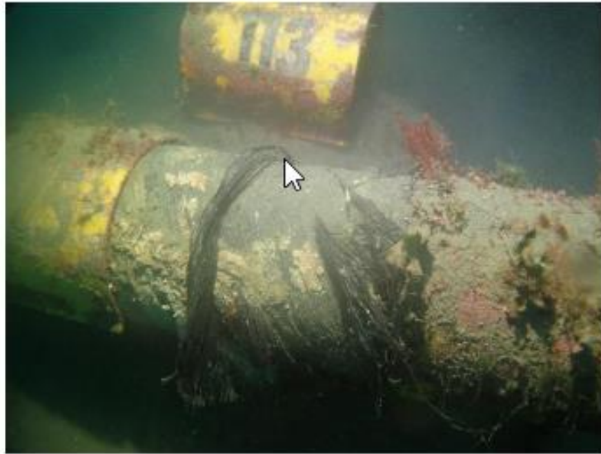
Figure 4: Armour exposure to underside of HVDC#4 KP0.575 beneath clip 113.
