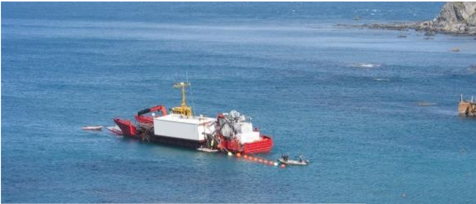
A barge laying a small section of submarine cable in Oteranga Bay in 2005 to complete a repair.
