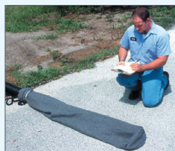
A filter bag can provide useful polishing and assurance of discharge of clean water from earthworks etc.
