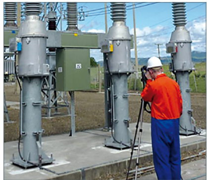
Using an SF 6 gas camera for leak detection.
