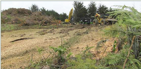
Mulching during vegetation clearance works to reduce sediment in run-off.
