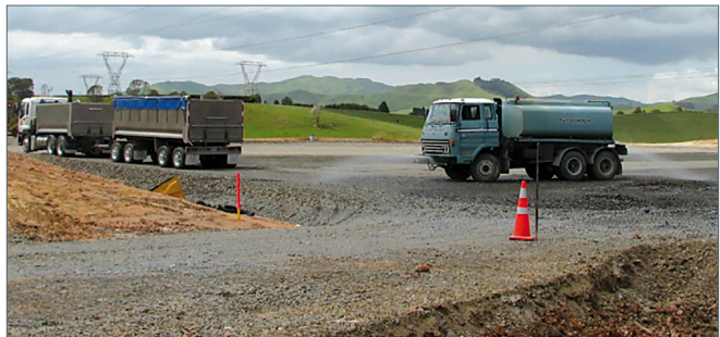
Use of a dust cart on a substation construction site.
