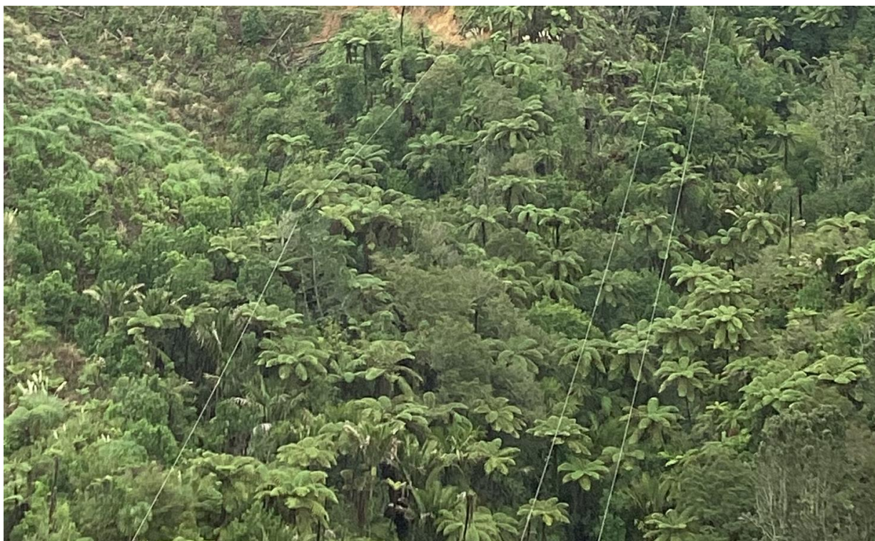
Figure 2: Span 107-108 of the EDG–WAI 2 circuit
